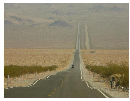
The vertical alignment or road profile is comprised of vertical curves and lines used to create crests, sags and tangents.
